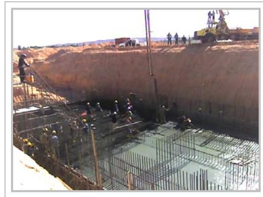
The project comprises construction of 3-7 meter deep concrete structures with 0.8m thick walls and spreading over an area of 30m x 18m.
